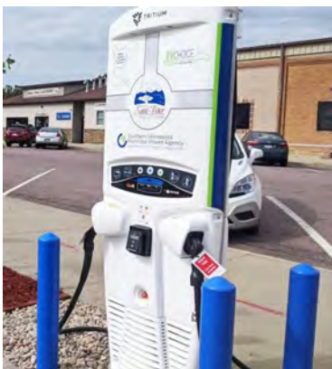
SMMPA's DC Fast Charger in Saint Peter
