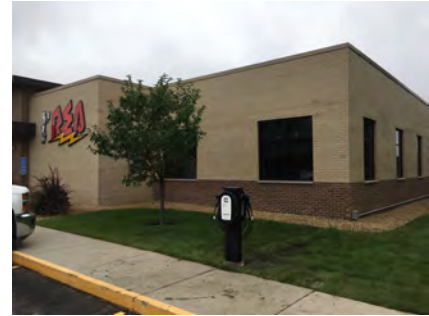
Runestone Electric Association Headquarters
